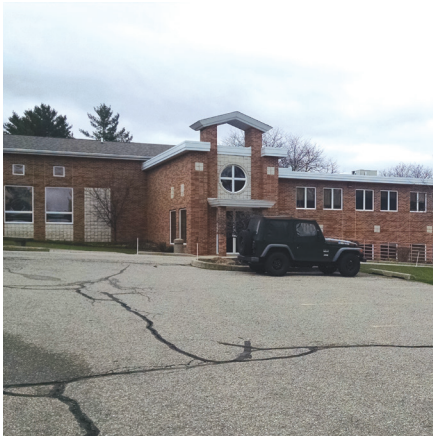
Cracks in Parking Lot
