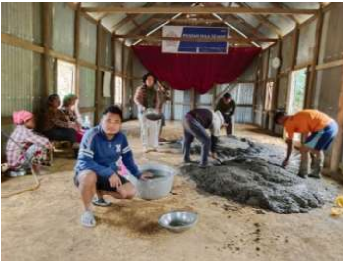
Installing floor at Kotlian Baptist Church
