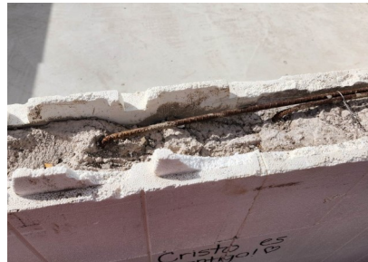
Styrofoam blocks, reinforced with concrete and rebar, are used for the foundation and walls. This results in a stronger, more enduring structure.
