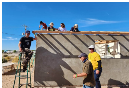
Getting ready to raise the roof.
