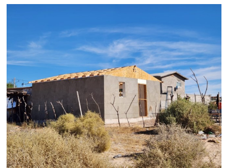
The trusses had been built by a prior group; it was our team's job to get them hoisted up and secured prior to adding the sheathing. Material.
