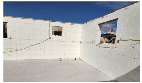
Channels are carved into Styrofoam for electrical wiring. The walls will be stuccoed.
